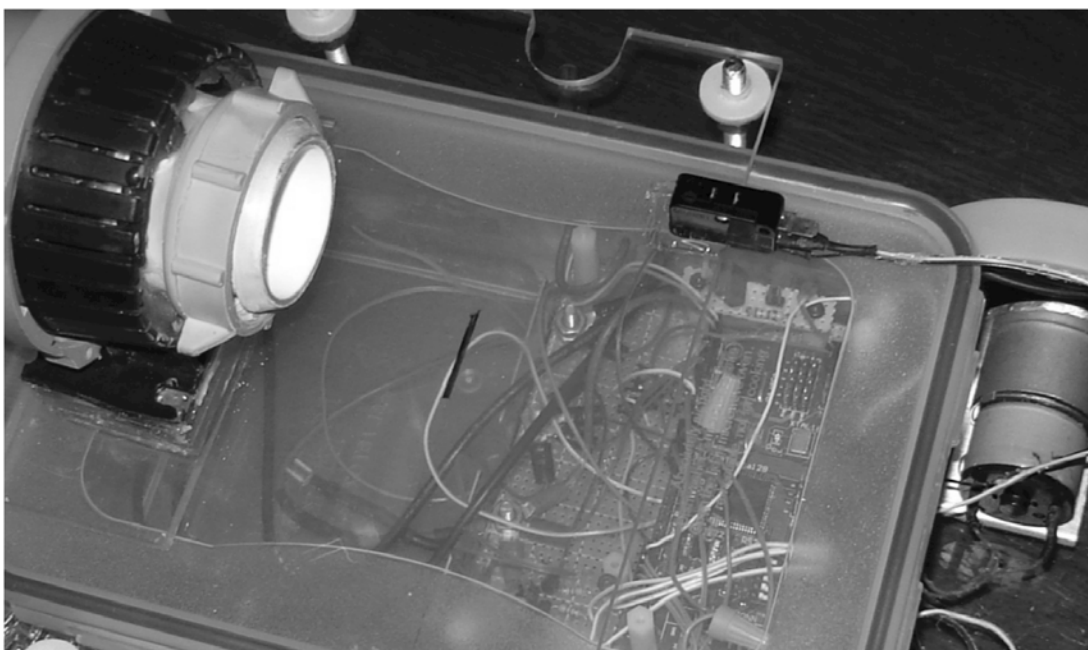
Figure 13. Momentary switch mounted to the top of the second tier to check for the bin
