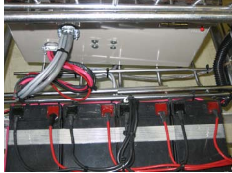
Figure 15 Data Lines along rail closest to Enclosure; Power is away
