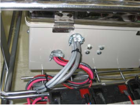
Figure 14 Sensor Enclosure; separate Data and Power
