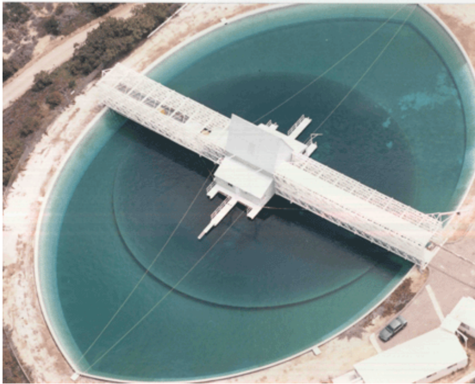
Figure 2: Aerial photo of facility. The water clarity shown is typical. The bridge structure has no piers or supports in the pond.
