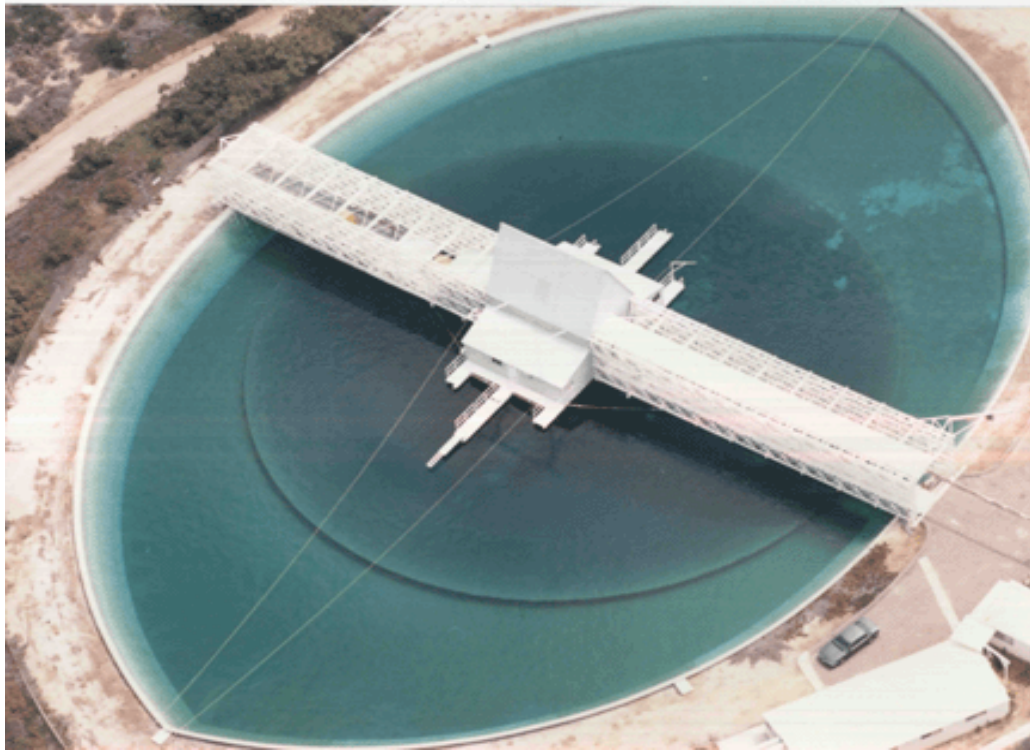
Figure 2: Aerial photo of facility. The water clarity shown is typical. The bridge structure has no piers or supports in the pond.
